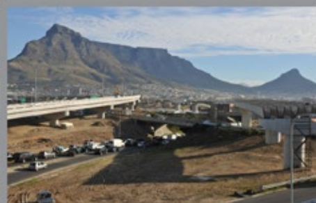
Koeberg Interchange, South Africa
