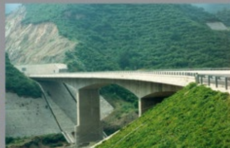
Badaling Expressway Overpass, China
