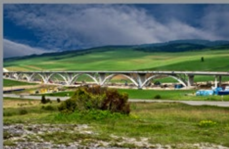
D1 Highway Bridge, Slovakia
