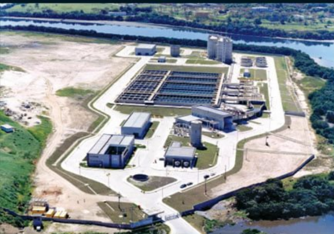
Allegria WWTP, Brazil
